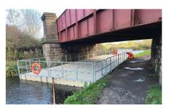
EZ Dock floating, modular dock systems are composed of two parts: polyethylene sections and moulded rubber couplers. Both components are made of materials that are completely harmless to the environment and can be recycled when the intended use is finished. EZ Dock provides more stability than traditional floating dock
